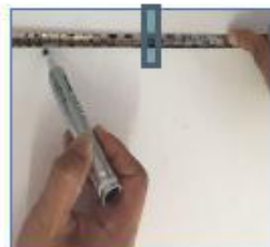
Mark the centre dimensions on the wall
