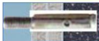
Insert the fitting into wall, leaving the thread exposed by 8 - 10mm
